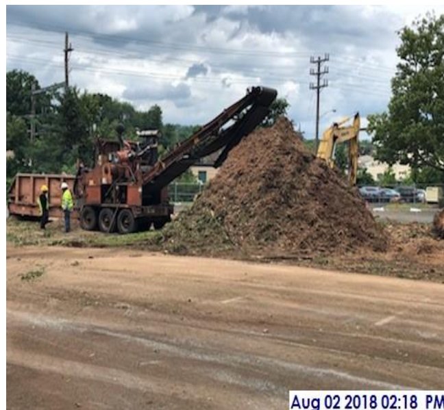
Mulch pile created from tree removal/chipping
