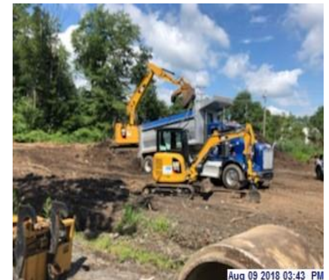
Grading & debris removal at New Salt Dome location
