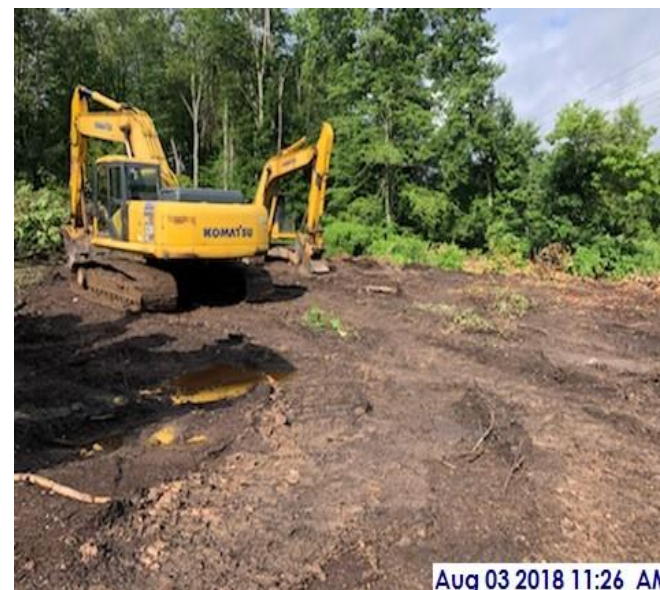
Site clearing at New Salt Dome Area
