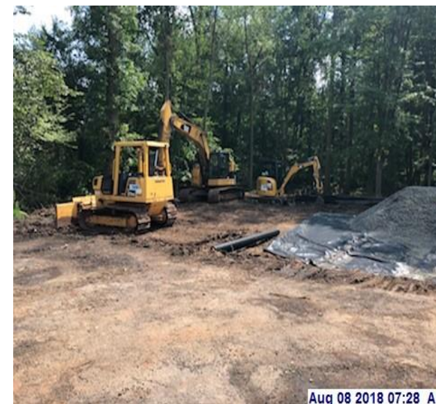
Grading adajecent to DPW garage for trailer pad
